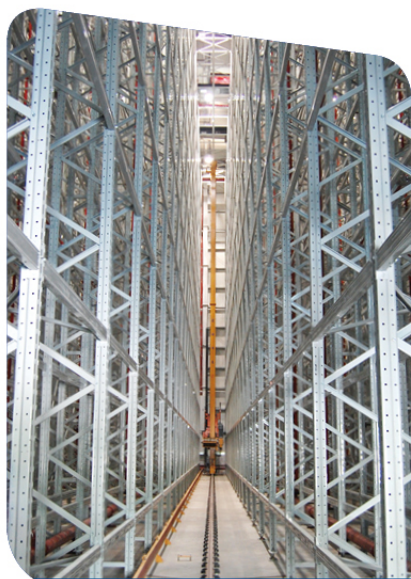
货架系统 Racking System
